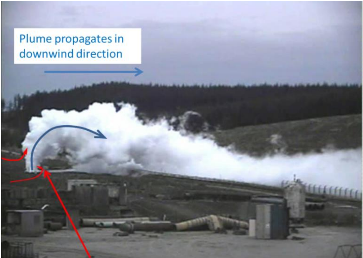
Fresh air entrainment possible around plume base
