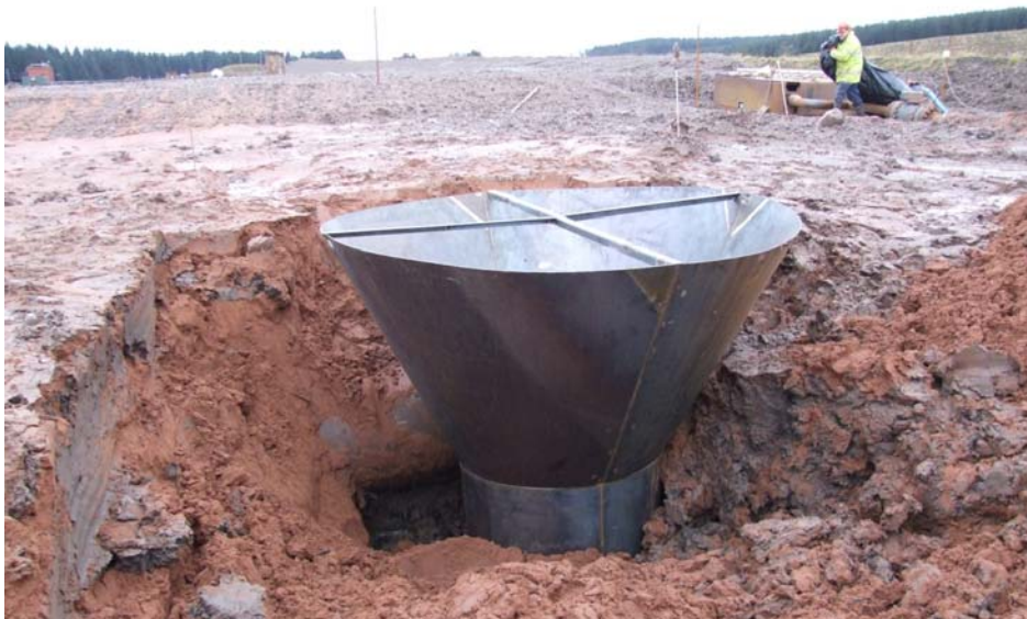
Figure 4 Pre-formed crater prior to burial
